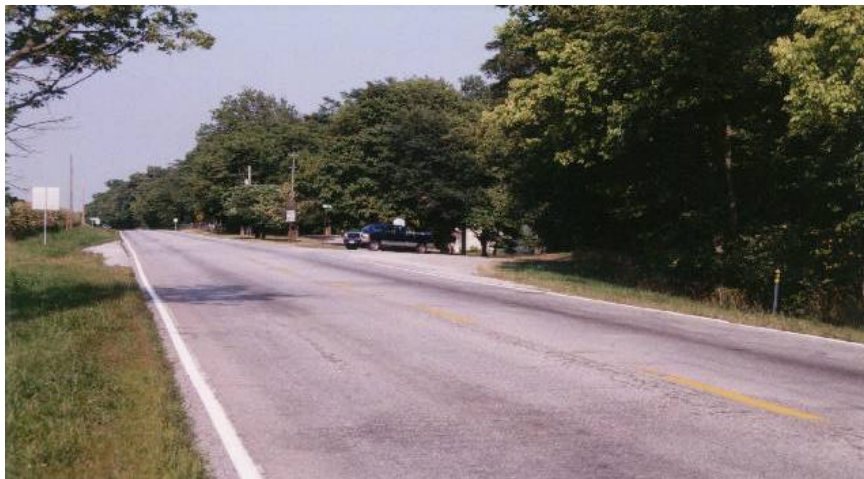
Figure 7: Intersection of SR25 and County Road 900N
