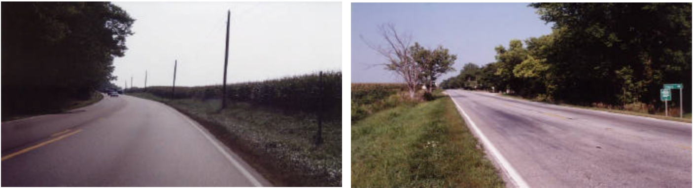
Figure 3: Typical roadside obstacle: Utility Poles and Trees
