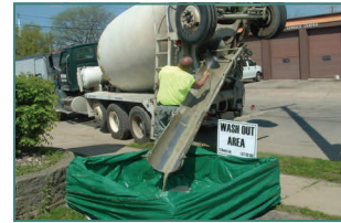
Vinyl washout container
