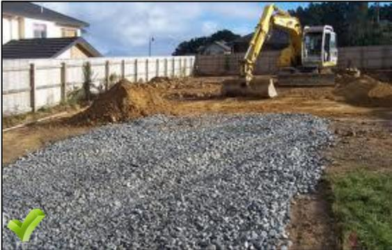
Each site should have a construction exit. A well-maintained construction exit keeps mud off the pavement and out of storm drains. If mud or soil is tracked on the road, it should be cleaned up immediately.
