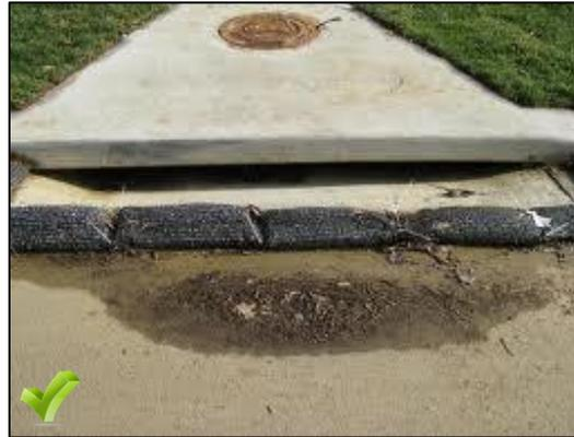
Provide inlet protection at curb inlets and/or catch basins around the building site. Never dispose of or deposit any substance into the storm collection system.
