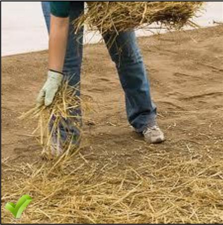
As soon as feasible, sites should be temporarily stabilized with straw, or permanently stabilized with grass and sod. When straw is used, it should be crimped or “punched” into the ground to prevent the straw from moving during wind and rain events. Erosion control mats or sod should be used in concentrated flow areas, such as ditches and swales.
