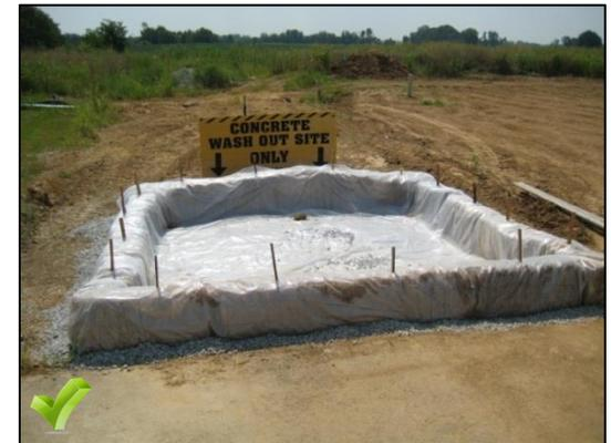
Contractors and subcontractors should utilize concrete washouts whenever pouring or placing concrete or mortar. Washouts should be used for rinsing off mortar and concrete mix, process and placement equipment. It is not acceptable to wash off equipment outside of a contained concrete washout area.
