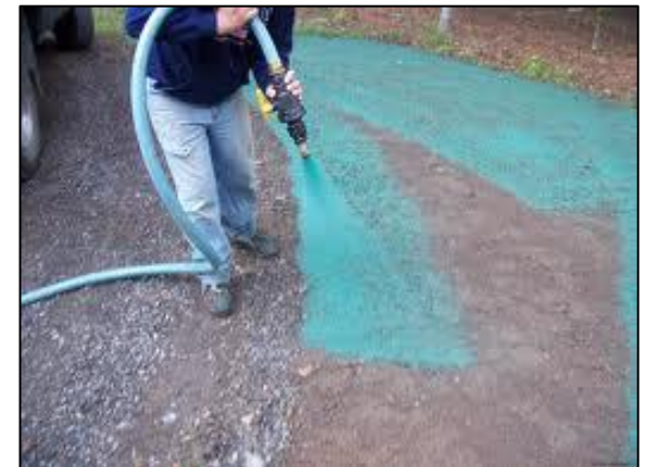
Hydro seeding applied to bare soil to speed up slope stabilization.
