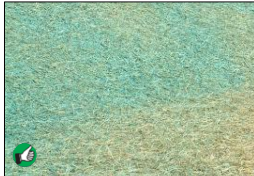
Straw applied evenly over newly seeded areas to provide temporary erosion control.
