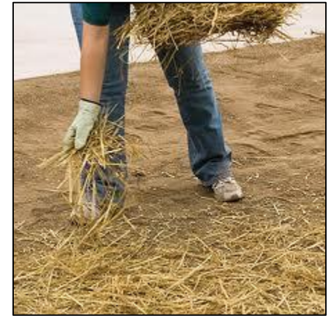
Straw mulch being placed by hand over bare soil.
