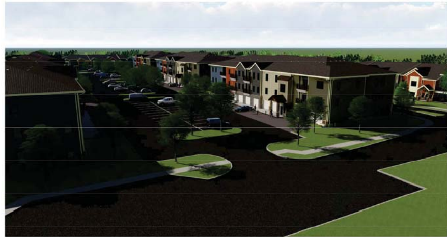
Precedent Flats Lafayette, IN Domo Development Company
